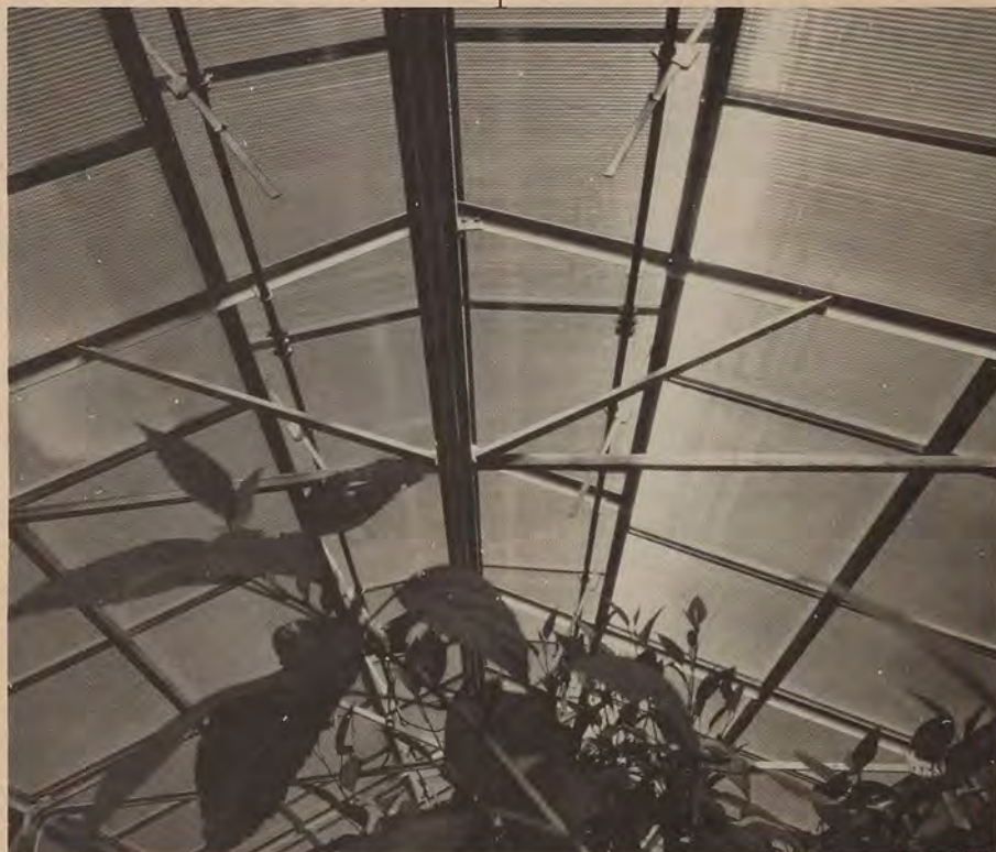
Acrylic's high strength and light weight permit installing the double-skinned sheets with supports on four-foot centers, which is not possible with single glass. Thus, installation cost is reduced as fewer structural supports are required.
